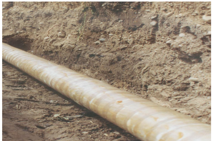
Section of 16" pipe reconditioned using #1 Wax-Tape.
